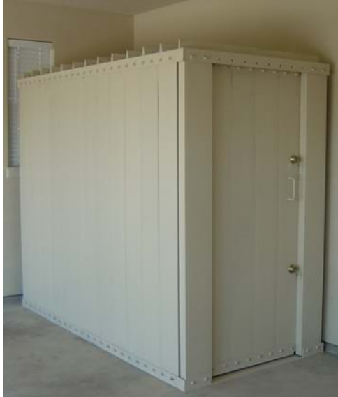
Figure 4: Engineers design secure structures to be placed inside an existing building. This interior room provides far more security in the chance of a tornado than the space around it.
